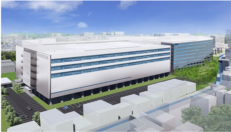
Yokohama Technology Campus Technology Development Building 이미지
